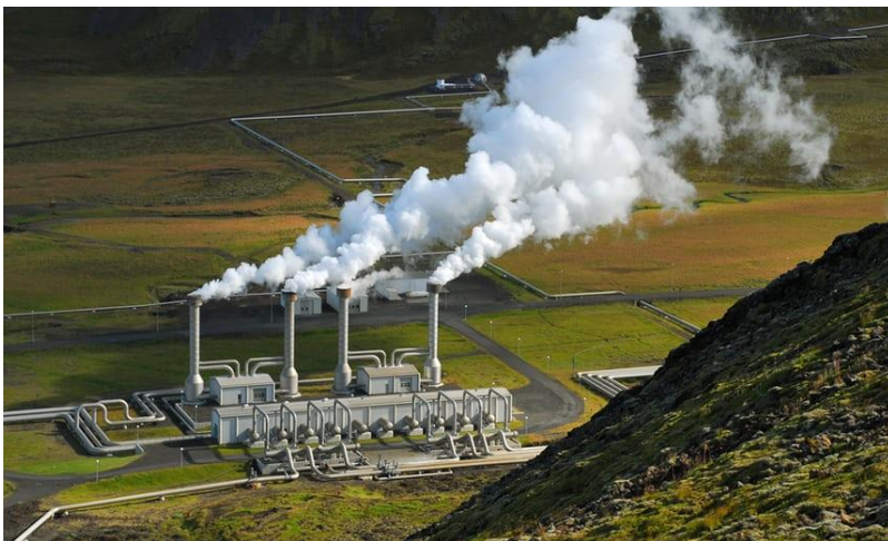
Fig. 28. The Nesjavellir geothermal plant in Iceland.
