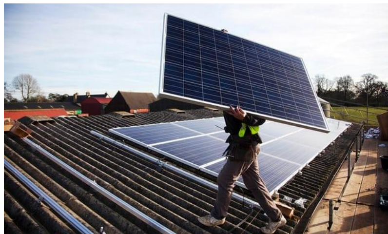
Fig. 20. Solar panel installation
